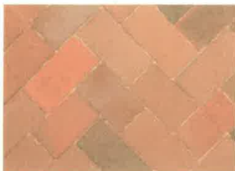
Picture 4: Double herringbone pattern using alternate 240mm and 200mm paviors
