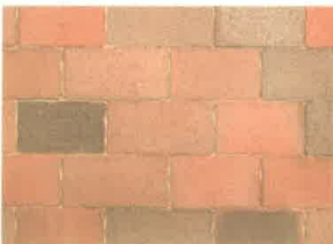
Picture 3: 'Flemish Bond' pattern using alternate 240mm and 200mm paviors
