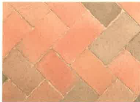
Picture 2: Herringbone pattern using alternate rows of 240mm and 200mm paviors
