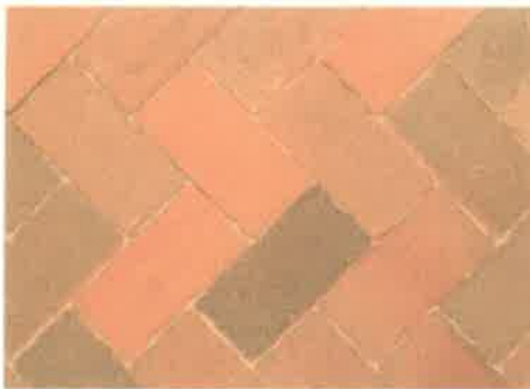
Picture 1: 45° herringbone pattern (240mm pavior only)
